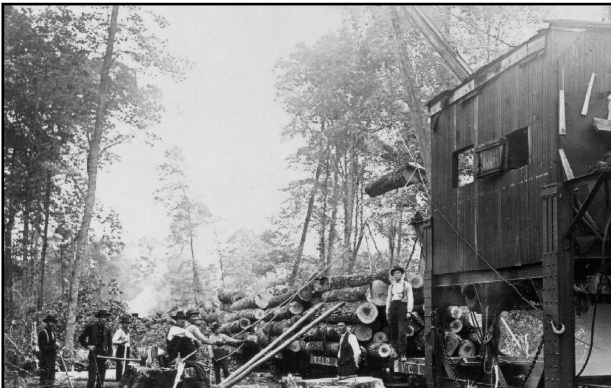
Photograph shows steel frame logging cars under a McGiffert Jammer.
