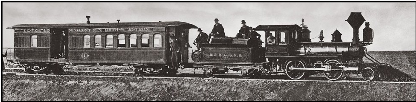
DL&NW Ry combine, half baggage and half passenger car pulled by a 2-4-0 "Porter" type Steam Engine.
